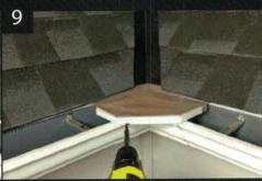
Test fit mesh for proper placement. Cut if neccessary.
